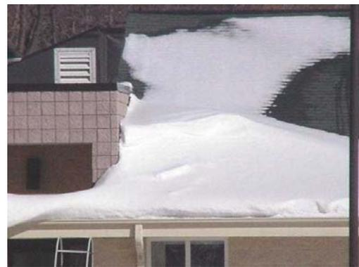
The heavy accumulation of snow on the roof could lead to the formation of an ice dam. Snow should be removed two to three feet from the roof edge.
