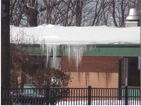
The formation of icicles is a good indicator that there is poor insulation/venting in the attic area. This can lead to water damage.
