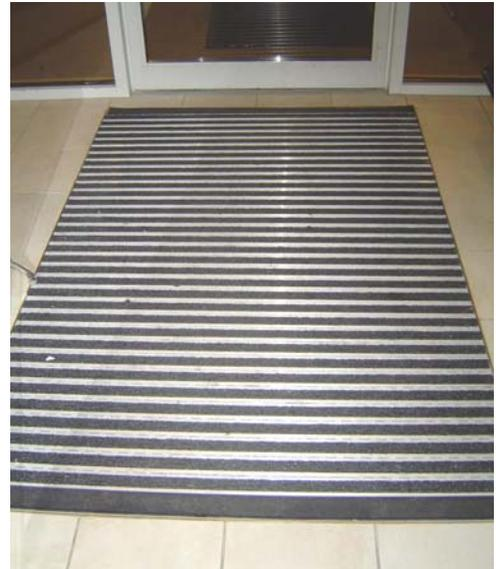
This photo shows an excellent control for minimizing the slip and fall potential in entryways. This is a grate system with a catch basin, which is built into the flooring surface. If this cannot be installed, use floor mats and/or runners.
