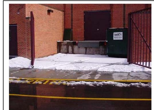
This photo illustrates how melting of snow from a loading dock can cause ice conditions to develop on walking surfaces.
