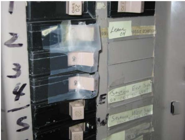
Image above shows breakers taped in the ON position. This practice should never be done.
