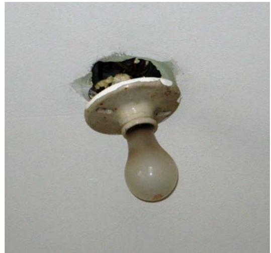
This image shows a light fixture that is unsupported, which puts undue stress on the electrical connections.
