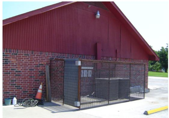
Example: This photograph illustrates AC units protected by a steel cage and security lighting.
